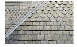
Slate shingles are fragile during installation and installers must be able to drive nails down to 1/8 inch above the shingle but no further.
