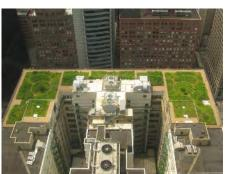
A vegetative roofing system also includes components like filters, a drainage system, and sometimes an irrigation system.
